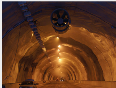
C-17 TUNNELS BARCELONA (SPAIN)
